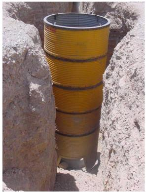
Photograph 3: Sample round manhole trench shield typically used during manhole installations (Courtesy: National Trench Safety website)
