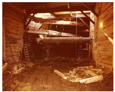
Photograph 1: 750 mm wastewater sewer through concourse during original construction in 1977 (Courtesy: City of Winnipeg)
