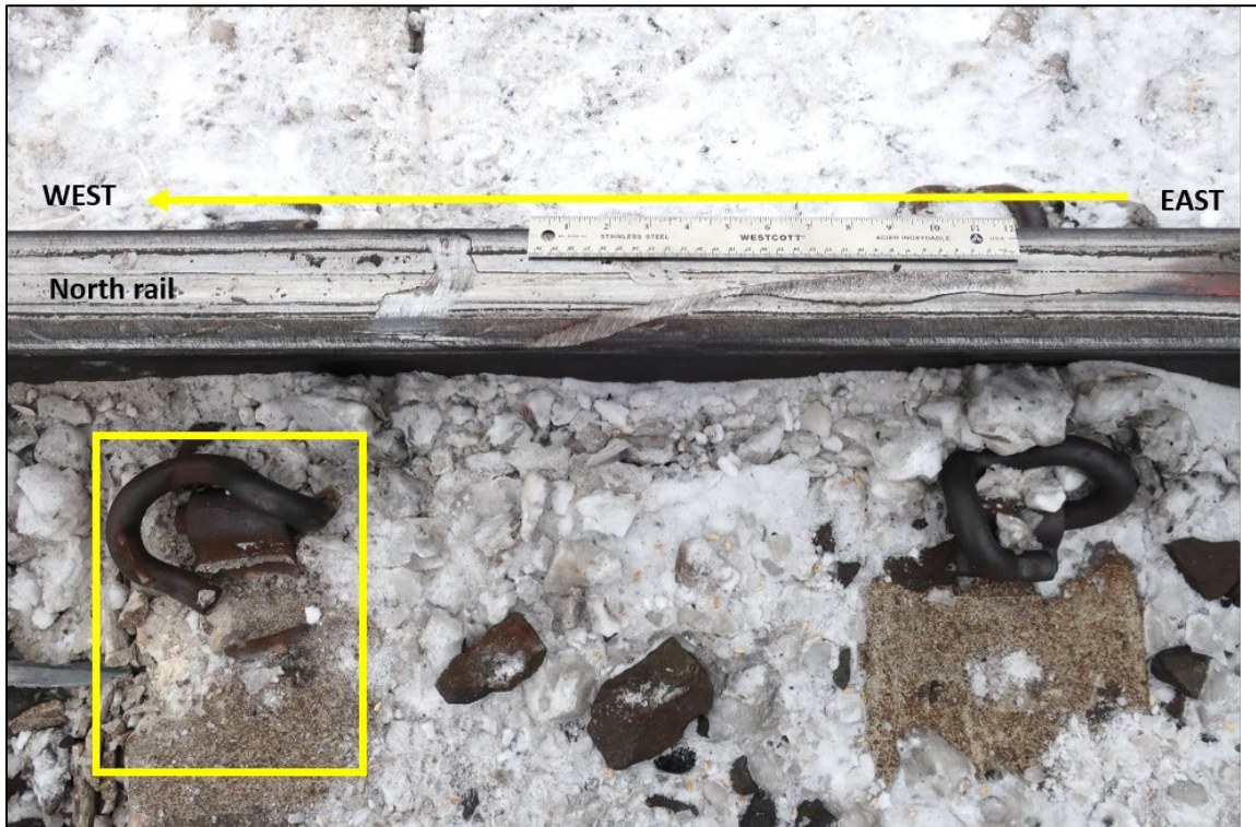
Figure 5. Wheel marks on the top of the north rail and the damaged gauge-side track fastener and tie (shown in the box) at Mile 166.33 (Source: TSB)
