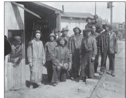
L.B. Foote with workers building tunnel under the Red River between Winnipeg and St. Boniface, 1918. N2378
